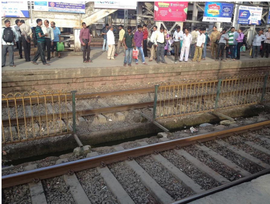
Opening in railing at Borivali Station
