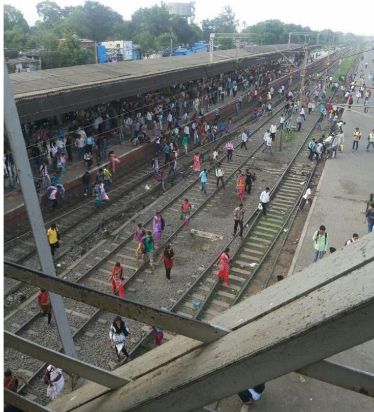
Lack of railings enables crossing of the tracks at Boisar Station
